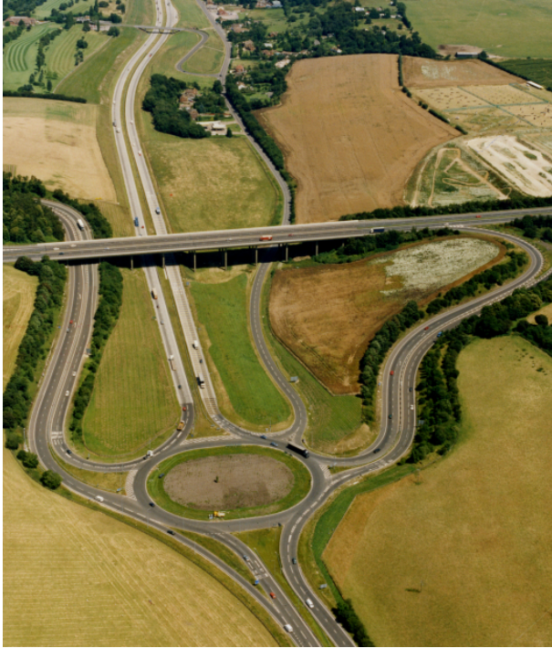
Picture 4.1.2 Junction 5 of the M2 with the A249
