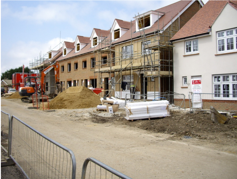
Picture 5.3.1 New house building in Faversham
